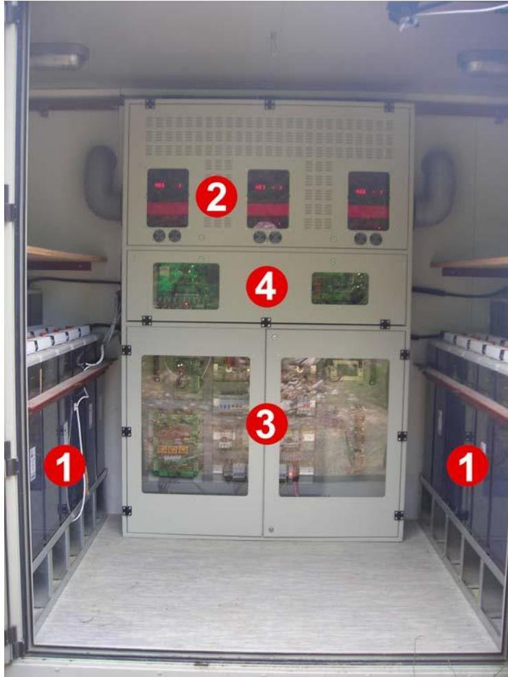
1. **A 48V Battery bank** (usually 1200 Ah capacity) **tubular OPZS open vent type**.
